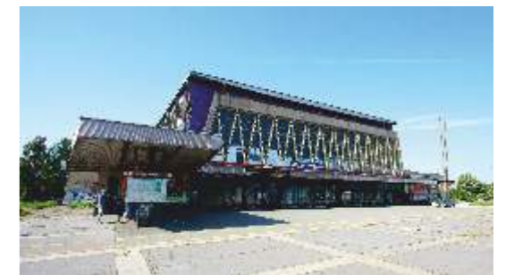
Railway Station Ostrava-Vitkovice
